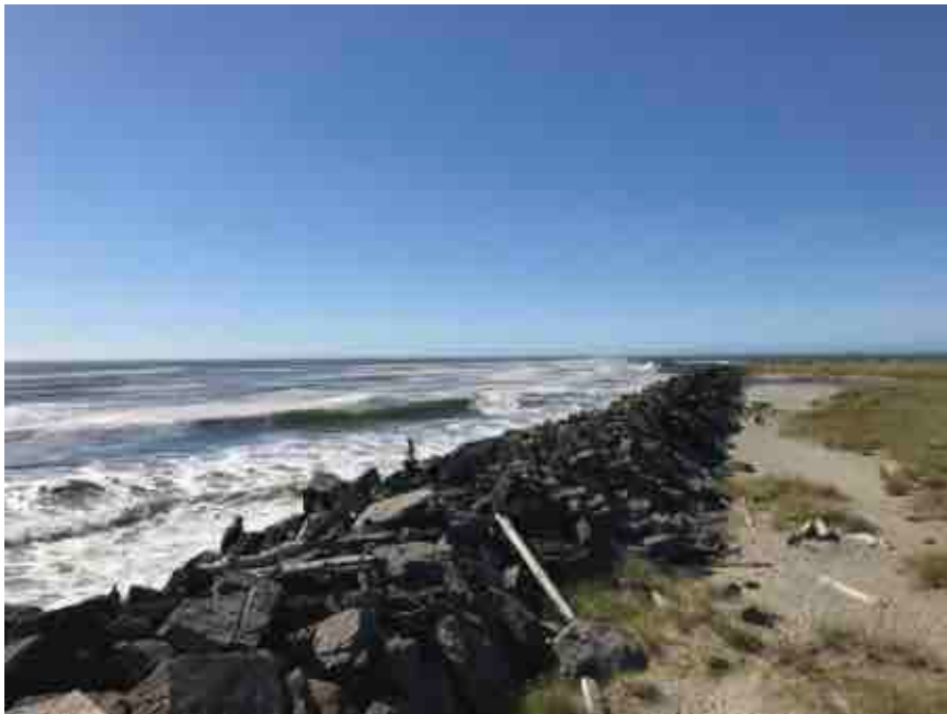
This jetty was built between 1885 and 1895. The jetties narrow the current to flush out sediment and help keep ocean beach sand from clogging the river's mouth.
